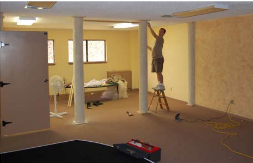
Pillars of Faith: Dan Giard puts the finishing touches on a column in the Master Peace Theatre.
